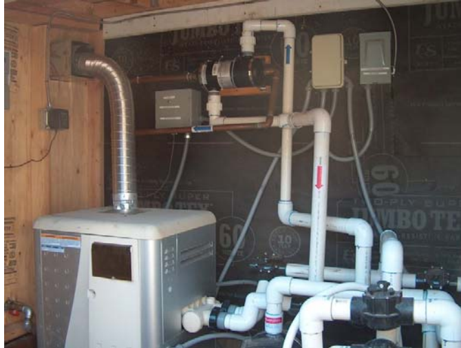
Picture 3: Tube-in-Shell Heat-Exchanger for Pool
