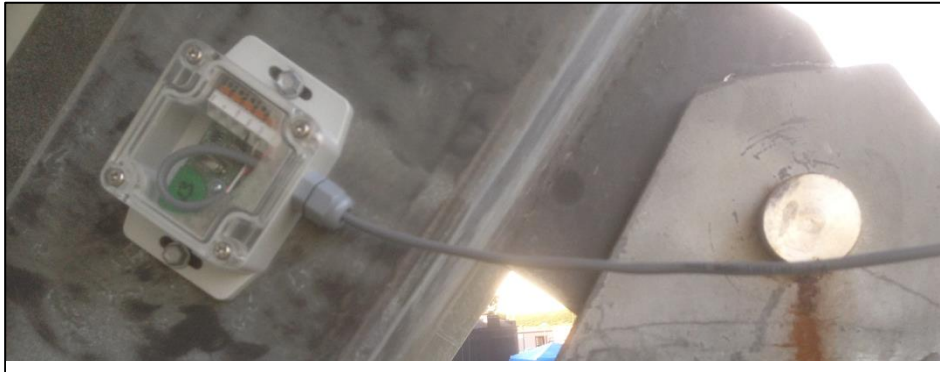
Figure 13; Positive oriented inclinometer on dual-axis tracker
